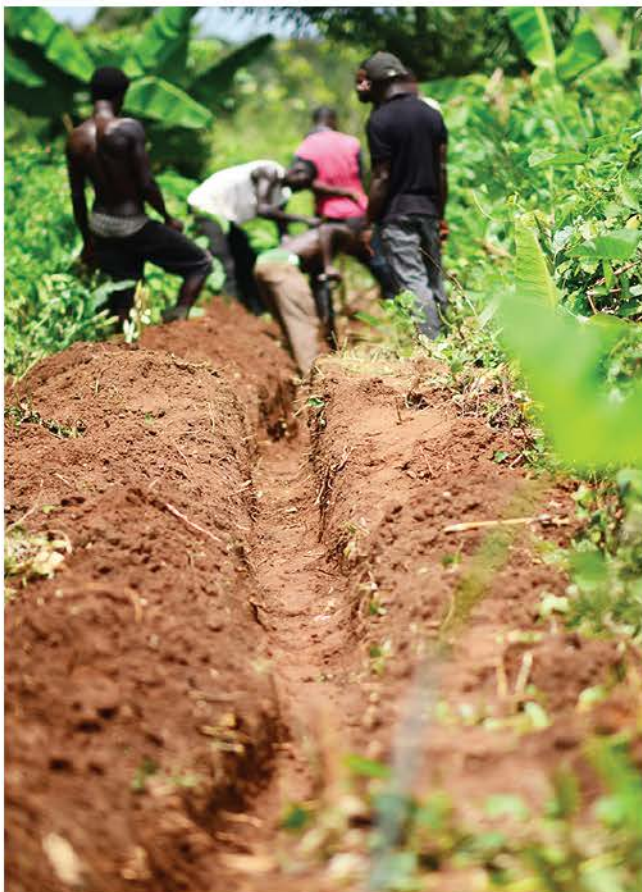
Trenches being dug for installation of pipe lines
